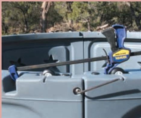
Wall panel tops held together with "QuickGrip" clamp and with Allen head bolt being installed.
